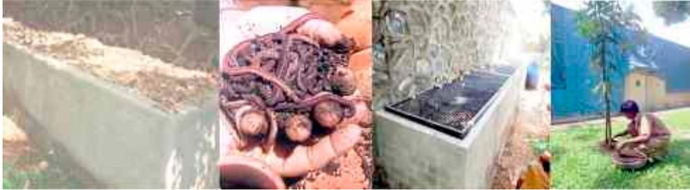
**Use of Organic Wastes Converter @ L-Center ,Banglore** - The Organic waste Converter was installed to to convert food waste into bio-fertilizer/manure. This manure is used within the campus for landscaping.
